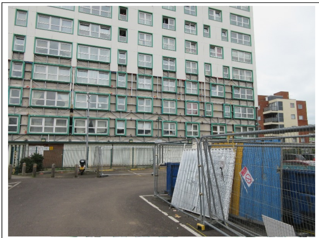
Figure 6 - West elevation, cladding removed to the 4 th storey
