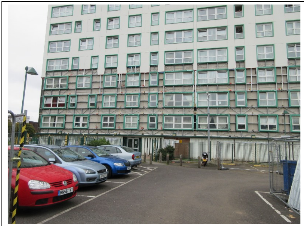
Figure 5 - West elevation, cladding removed to the 4 th storey
