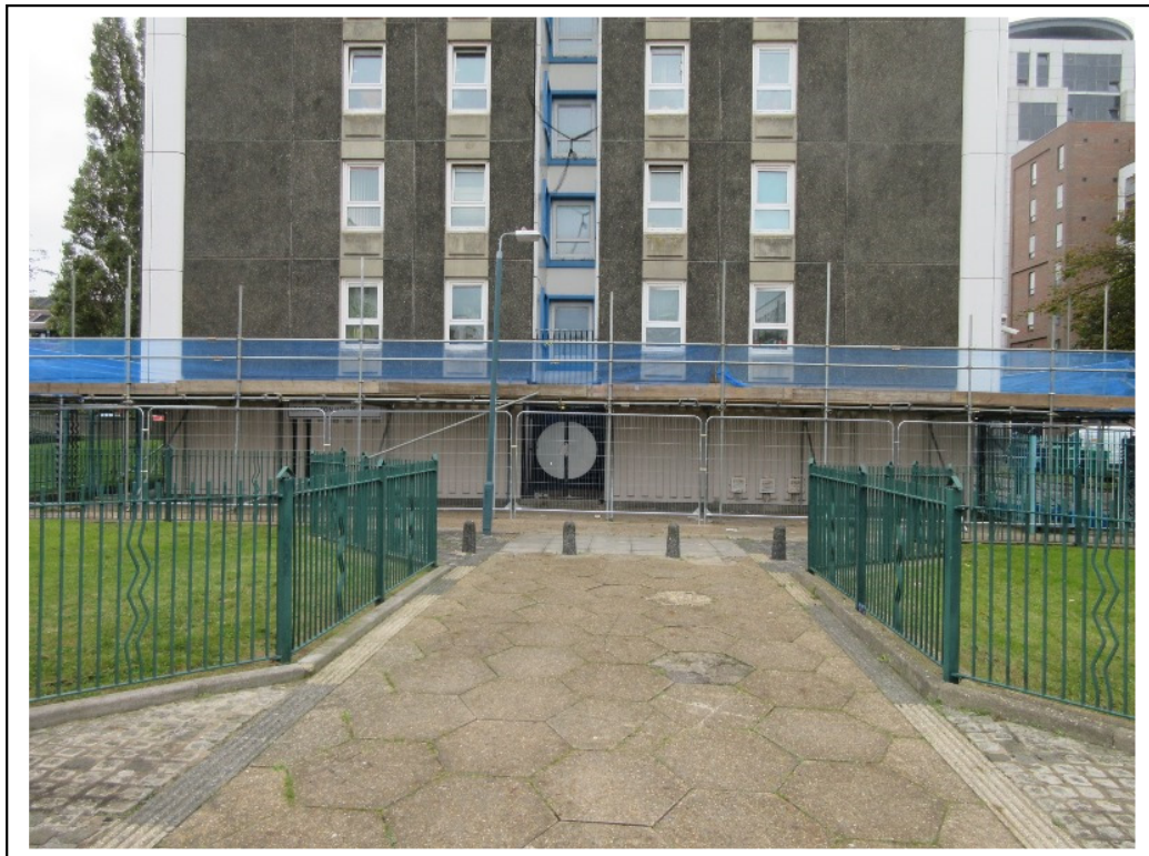
Figure 16 - Scaffold fan installed to south elevation
