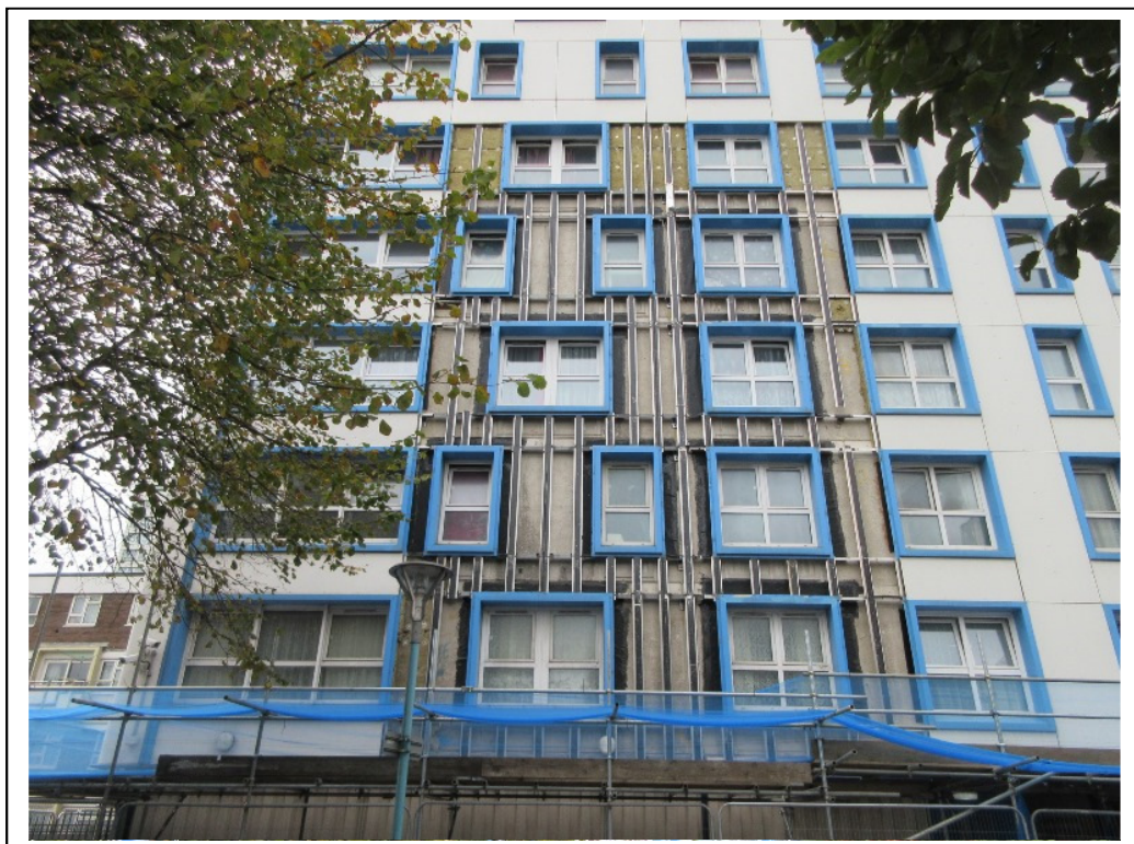
Figure 12 - East elevation, cladding partially removed to the 5 th floor
