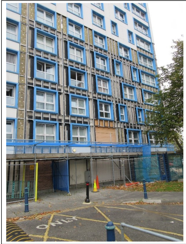
Figure 13 - East elevation cladding partially removed to 5 th floor
