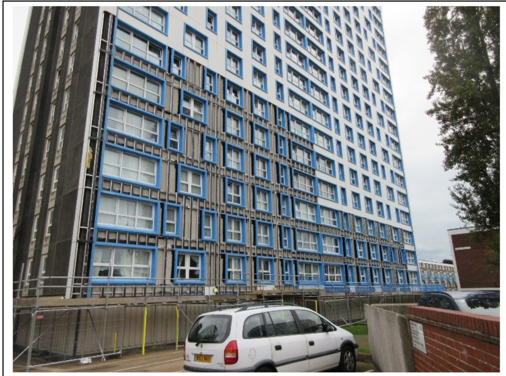
Figure 14 - West elevation, 50% of cladding removed to 7 th storey, remainder of cladding removed to 4 th storey
