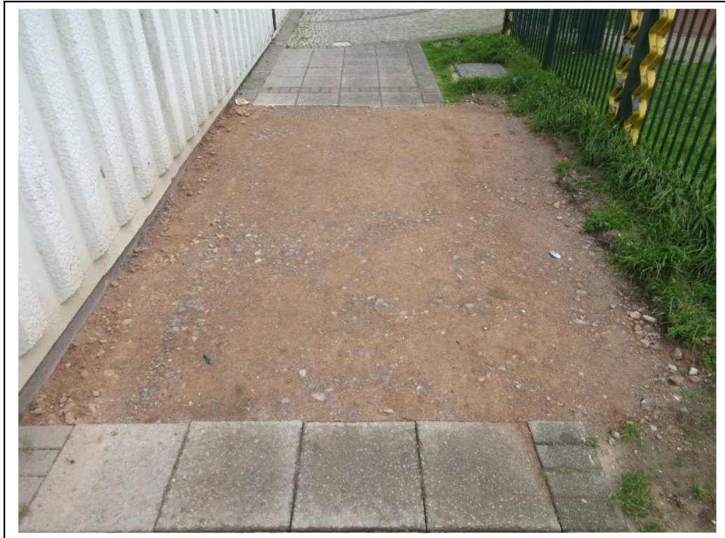
Figure 7- Example of a completed foundation to enable the mast climber installation
