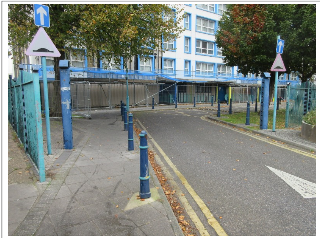
Figure 11 - Scaffold fan erected to main entrance, east elevation
