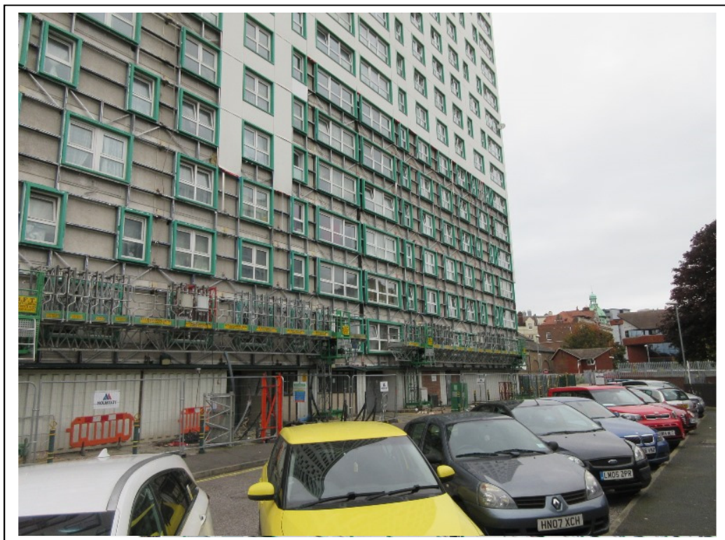
Figure 2 - East Elevation cladding removed to 6 th floor, mast climber installed to 1 st floor level
