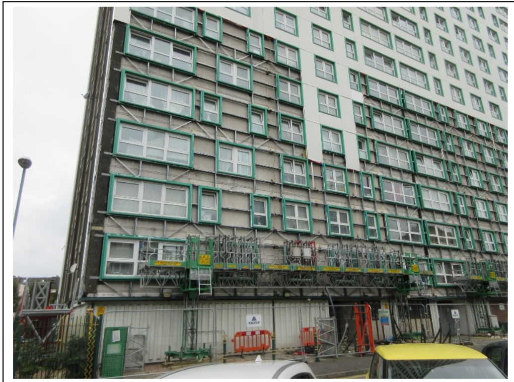
Figure 1 - East Elevation cladding removed to 6 th floor, mast climber installed to 1 st floor level
