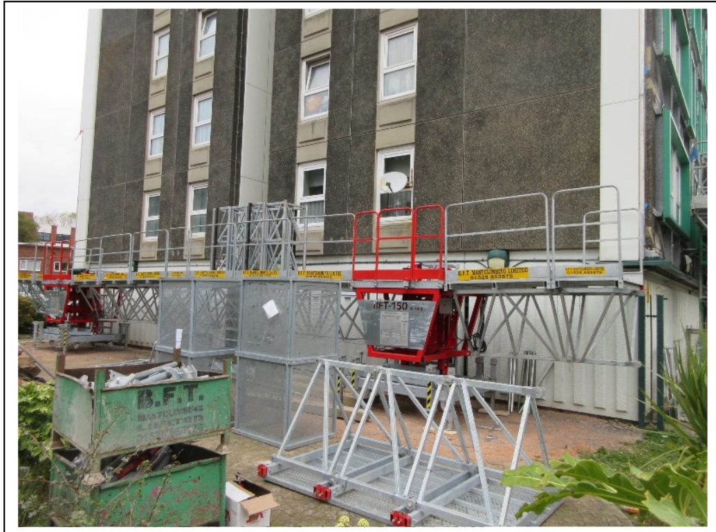
Figure 3 - Mast climber being installed to south elevation
